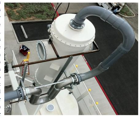
the contaminants are absorbed into the scrubbing liquid, the moist air is then directed through a mist eliminator to remove the droplets within the airstream, then the cleaned gas is discharged to atmosphere.
